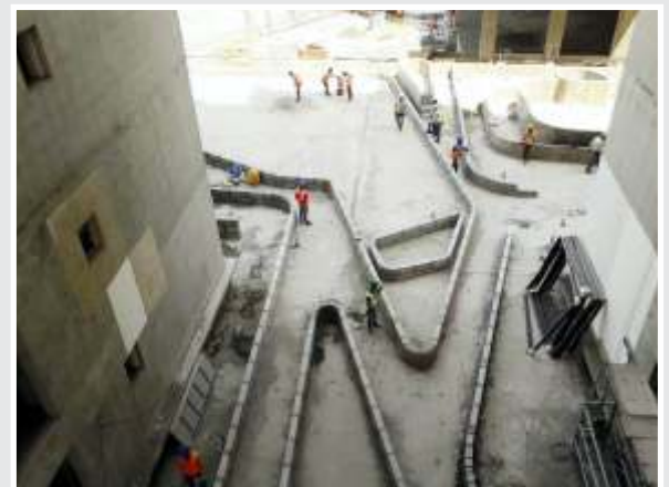
The Landscape Podium work-in-progress
