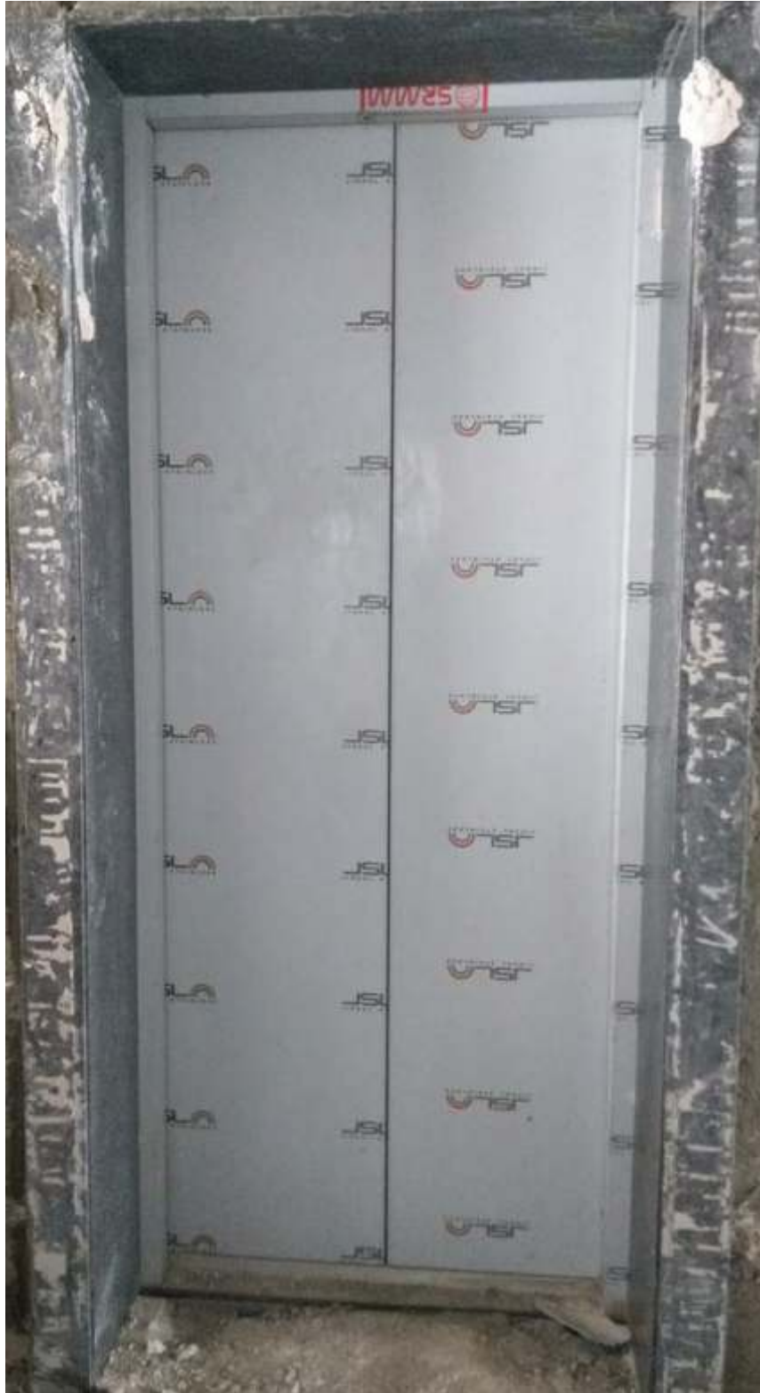
Lift Granite work in progress
